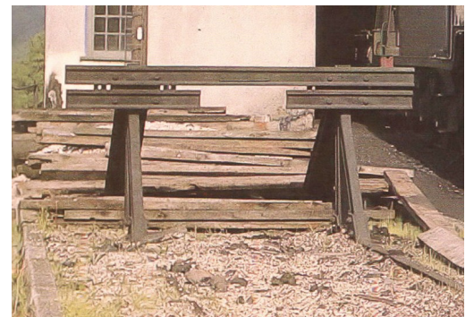
Buffer stop with gap in lower rail. Okehampton, 1960.
