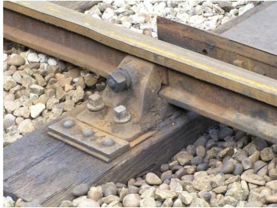
Fig 1 Prototype Joggle (Also note the bolted chair always used for switch chairs both BH and FB because there is nothing to restrain the rail on the inside)
